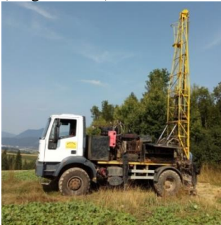
Figure 3: Core-drill rig at Site 2 (August 2018)
